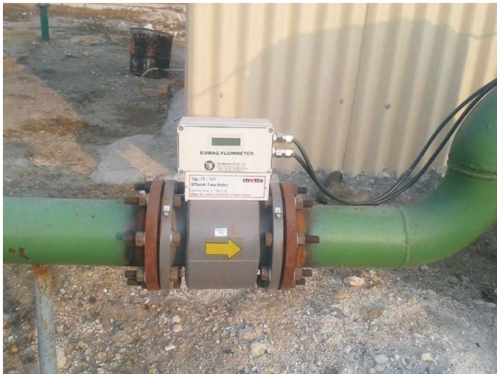
Flow meter for outlet Treated Water
