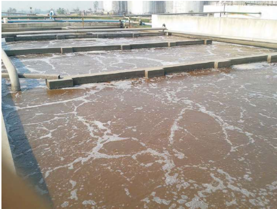
Old diffuse aeration tank
