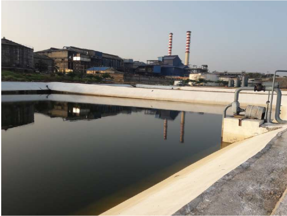
15 Days Storage Tank-1
